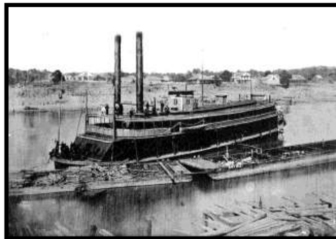
USS Forest Rose assisting construction of Bailey's Dam, May 1864
