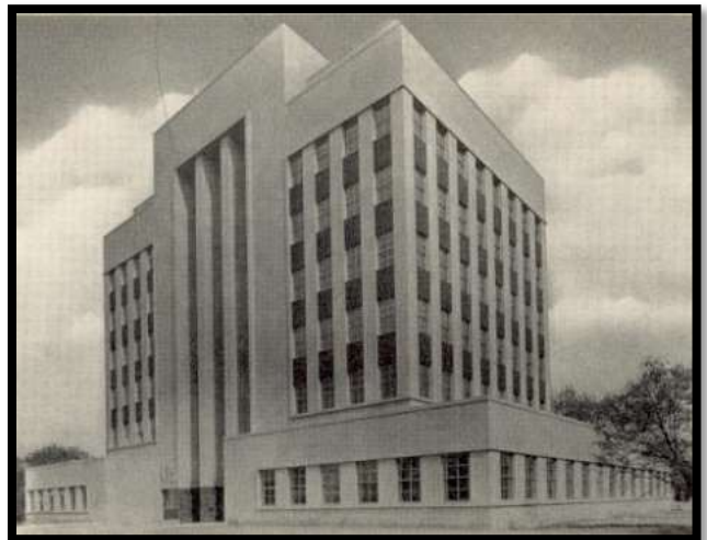
Rapides Parish Courthouse 1939-Present
