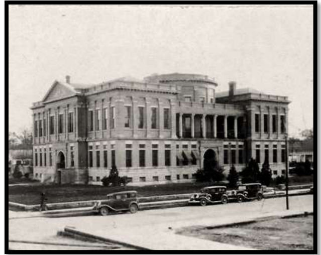
Rapides Parish Courthouse 1903-1939
